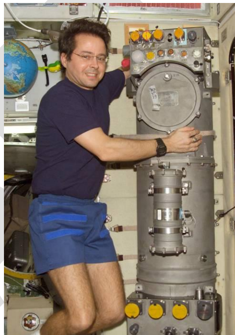
Figure 3: Astronaut Daniel W. Bursch working on the Elektron Oxygen Generator in the Zvezda Service Module on the ISS
